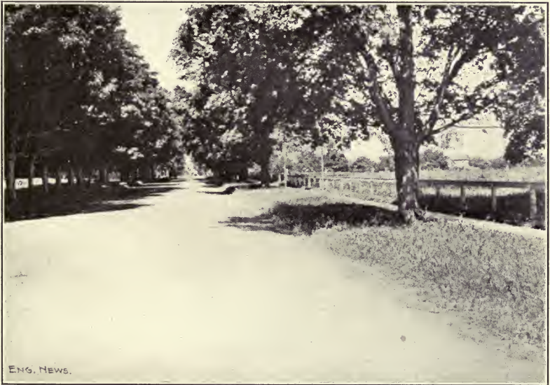
FIG. 8.—MACADAM ROAD WITH SHALLOW DITCHES, AFTER WINTER'S USE.
